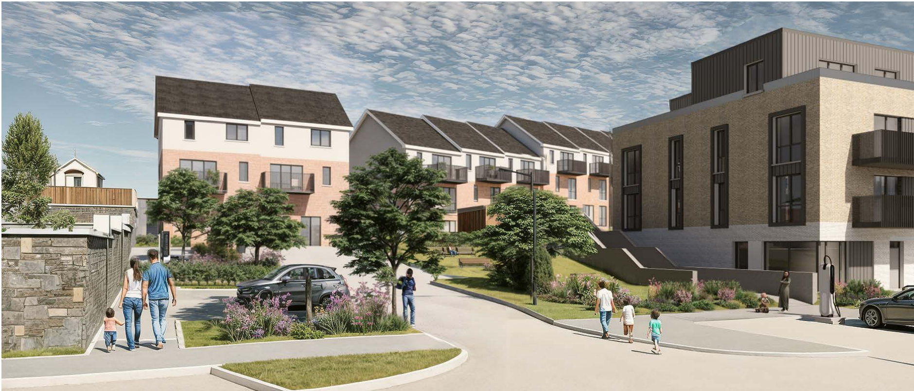
Fig 2B.1 (View 4) Image looking at area to the Rear of Units 1-6
